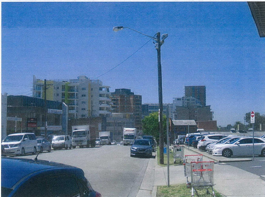
Figure 10: View of the frontage of the car park to Treacy Street looking east
